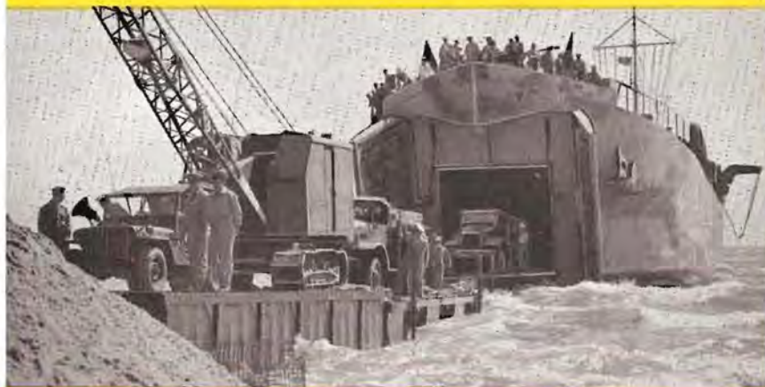
● As part of advanced training at Port Hueneme, Calif., Seabees receive intensive training in landing operations. Equipment is being unloaded over a pontoon causeway from the LST.
