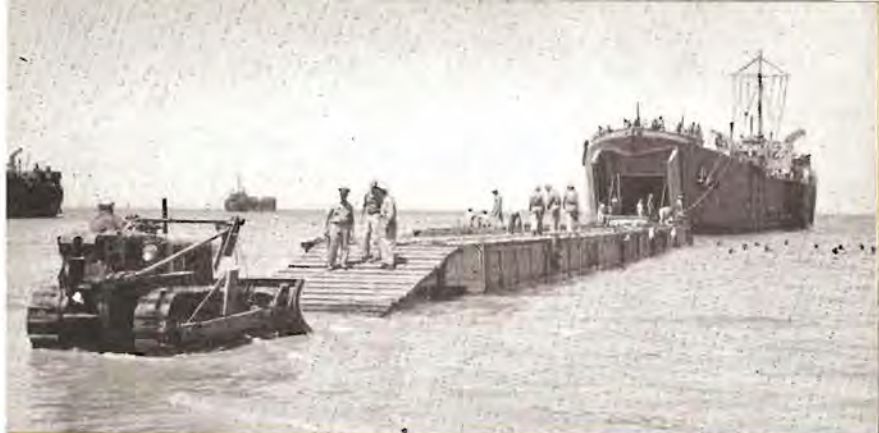
● On the beach at Sicily. Seabees run a bulldozer ashore over the pontoon causeway from the LST. Other Seabees unconcernedly are swimming alongside the landing craft.
