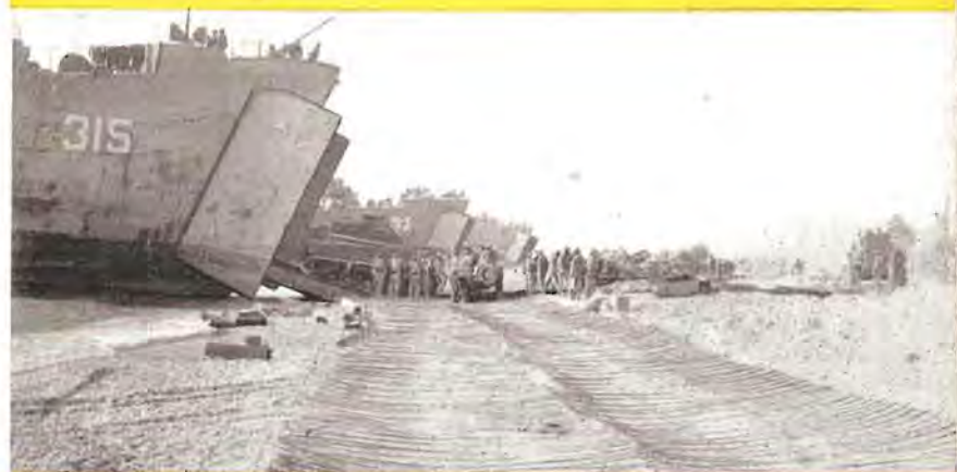
● Salerno, Italy. Seabees unloading Army tanks from an LST. Wire mesh has been laid over the soft sand on the beach so that vehicles may proceed quickly to the front lines.
