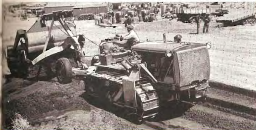
● Seabees use heavy equipment in the Aleutians to build the landing fields, docks and encampments for the Army, Navy and Marines.
