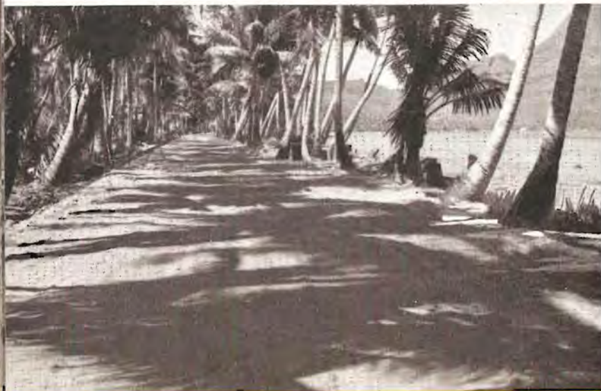
● Before and after. The upper picture shows the beginning of a roadway along the beach; and below, the park-like drive which appeared in a few days.
