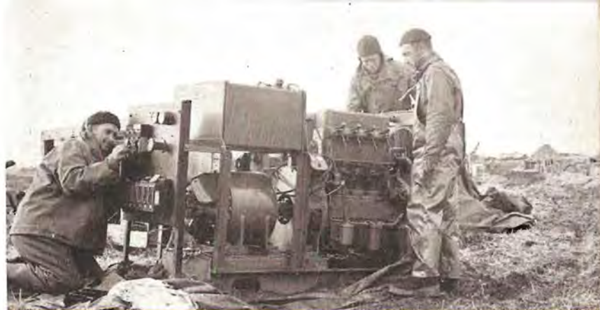
● On an Aleutian beach Seabees set up a Diesel Electric Generator as quickly as possible after landing in order to supply electric power.
